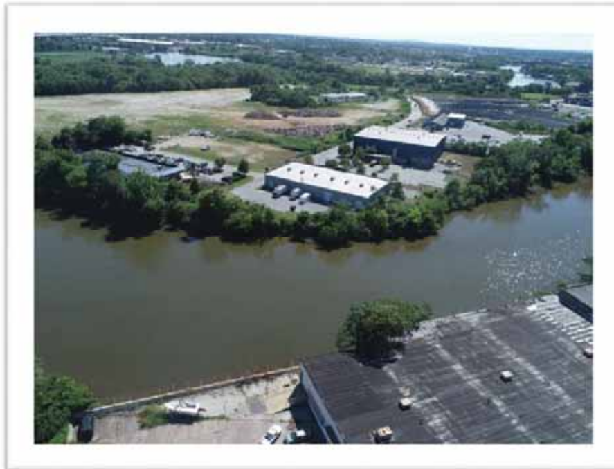
Looking West toward Wilmington Industrial Park from Across Brandywine Creek
