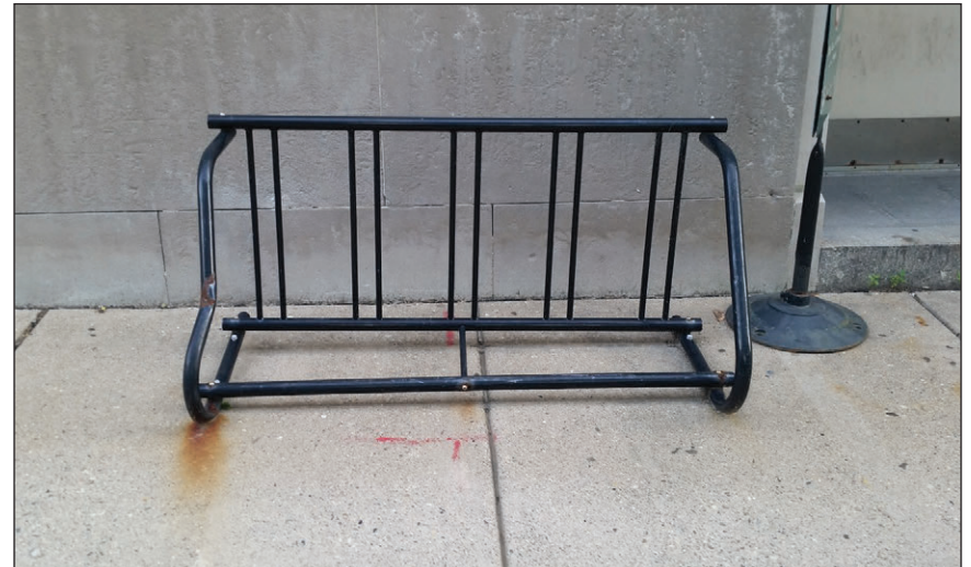
FIGURE 8: BIKE RACK STYLE TO AVOID GRID BIKE RACK LOCATED TOO CLOSE TO A WALL
