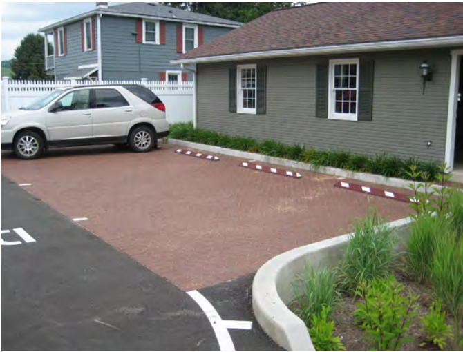
Permeable Paving and Gray Water Capture, Retention, and Park Irrigation System.
