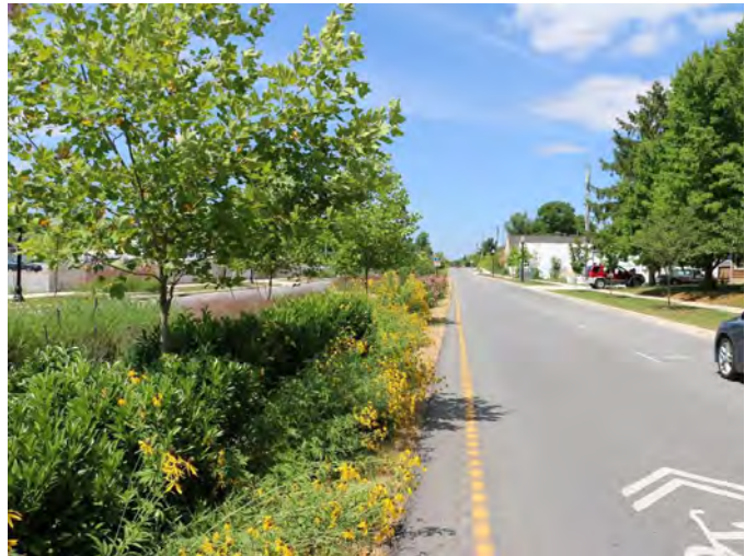
Micro-Pool Stormwater Swale.
