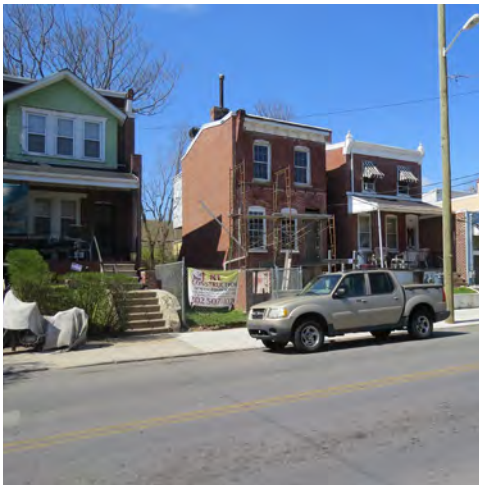
Homes being rehabbed along Vandever Avenue.
