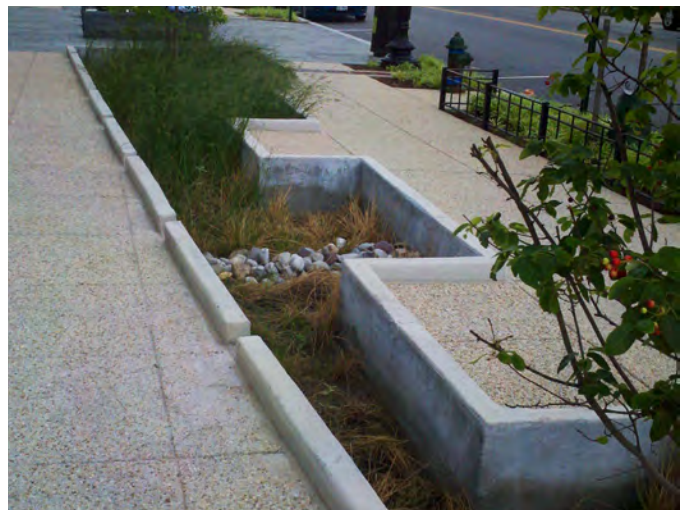
Bio-Filtration Stormwater Swale and Plazas.
