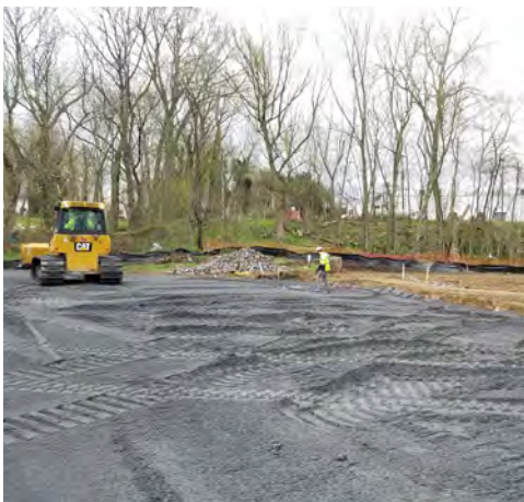
Site preparation of brownfields performed in accordance with regulatory requirements.
