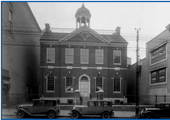
Old Town Hall, 504 Market Street, c. 1927; Market Street C.H.D. Courtesy of the Historical Society of Delaware.
