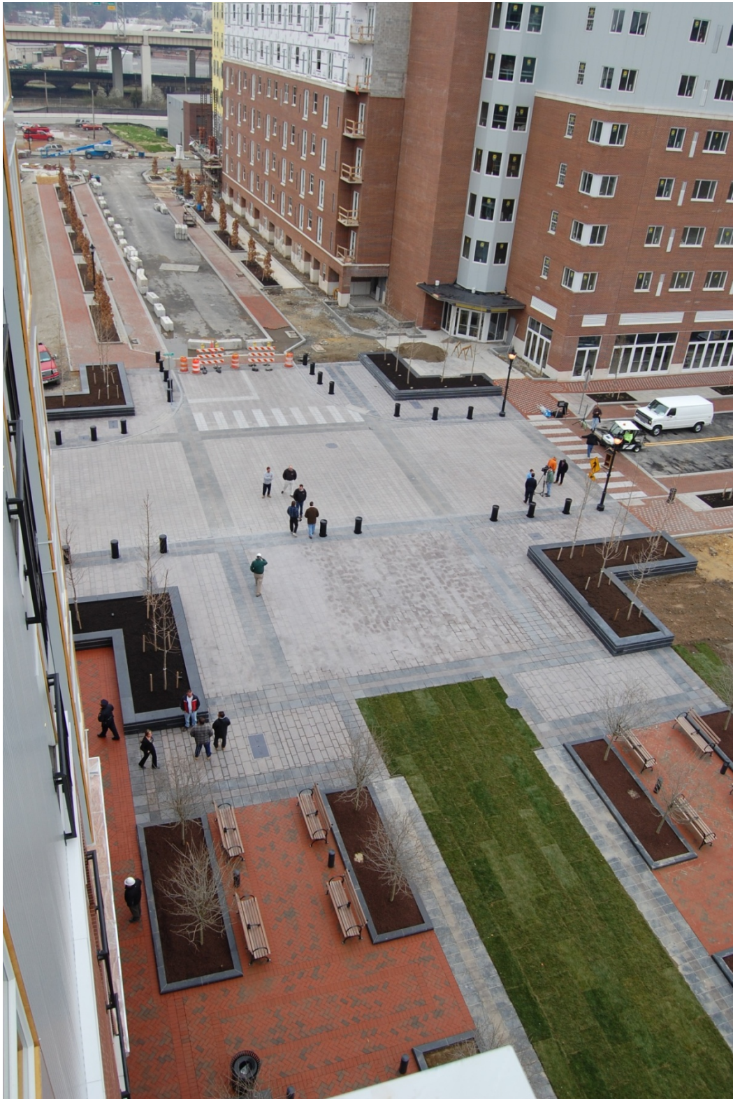
Work in Progress at Justison Landing
