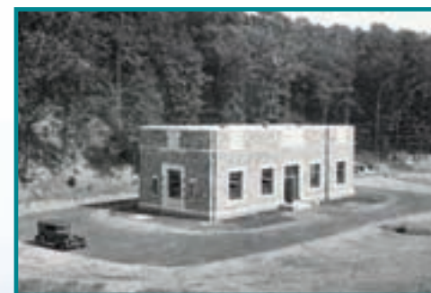
A pumping station with 3 gasoline-engine-driven centrifugal pumps was constructed at the base of the dam.
