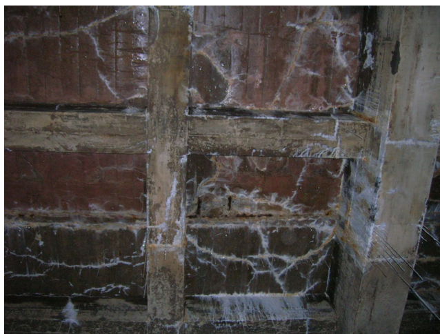
Spalled concrete exposing corrosion of the reinforcing steel Note: construction joint provides path for water / anode formation Gredell & Associates, 21 September 2006
