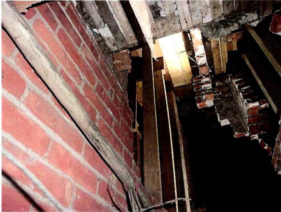
Photo 1 – Alley between 816 and 818 N. Adams Street
