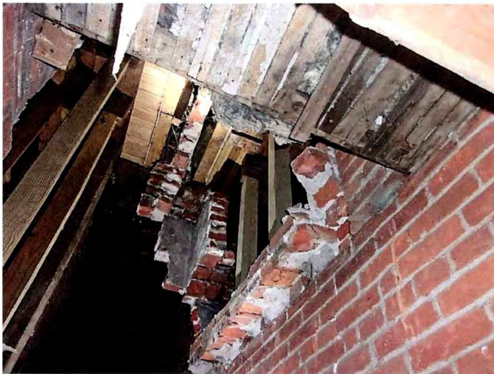
Photo 2 – Alley between 816 and 818 N. Adams Street
