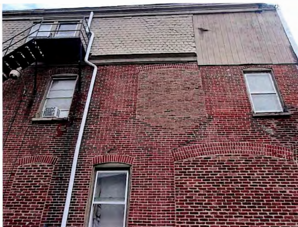
Photo 8 – Wall displacement/cracks
