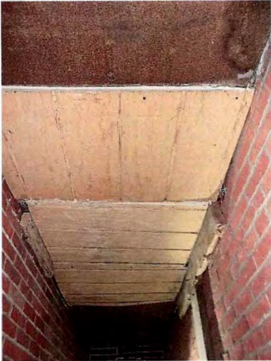
Photo 12 – Existing wood panels above alley at 812/814 N. Adams Street
