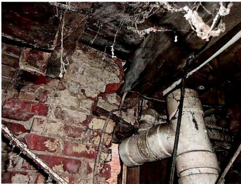
Photo 13 – Unsuitable wall bearing below floor joist
