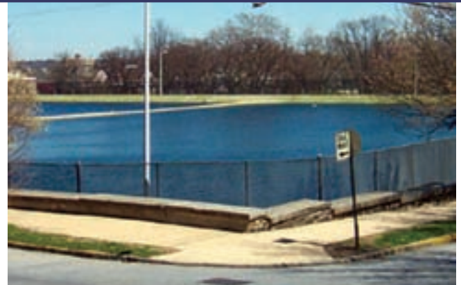
Current View of Cool Spring Reservoir which will be redesigned using an underground holding tank.
