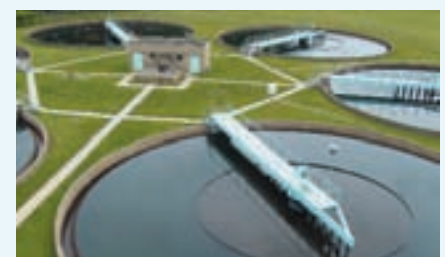
Porter Filtration Plant
